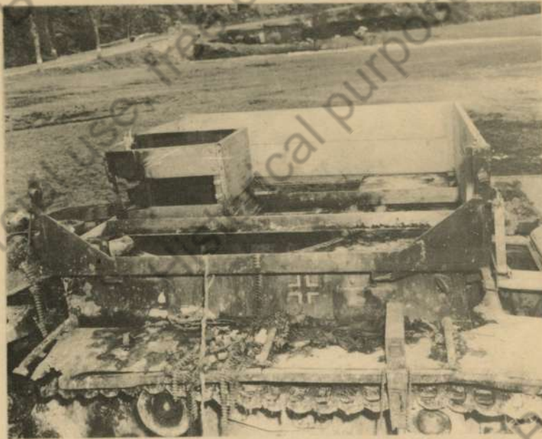
Figure No. 2: Close-up of box showing construction. Note attachment of longitudinal pieces to turret ring.
