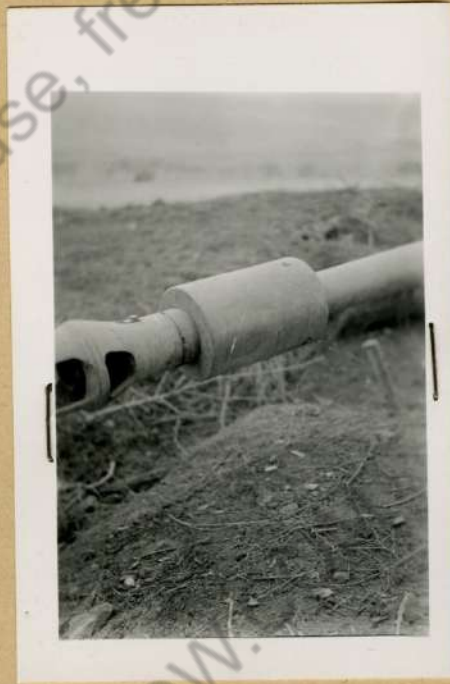
Photo No. 12 View of counterweight at muzzle end of tube. Note position in relation to muzzle brake.
