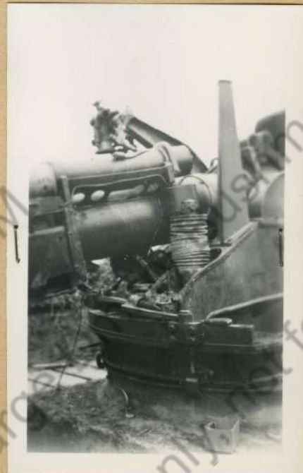
Photo No. 10 Right front view showing leather "shoe" at front of pedestal and concrete base into which base ring is set. Note bearing surface of rebound clip at rear of pedestal.
