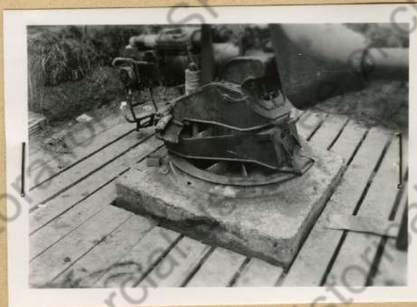
Photo No. 10 Right front view showing leather "shoe" at front of pedestal and concrete base into which base ring is set. Note bearing surface of rebound clip at rear of pedestal.
